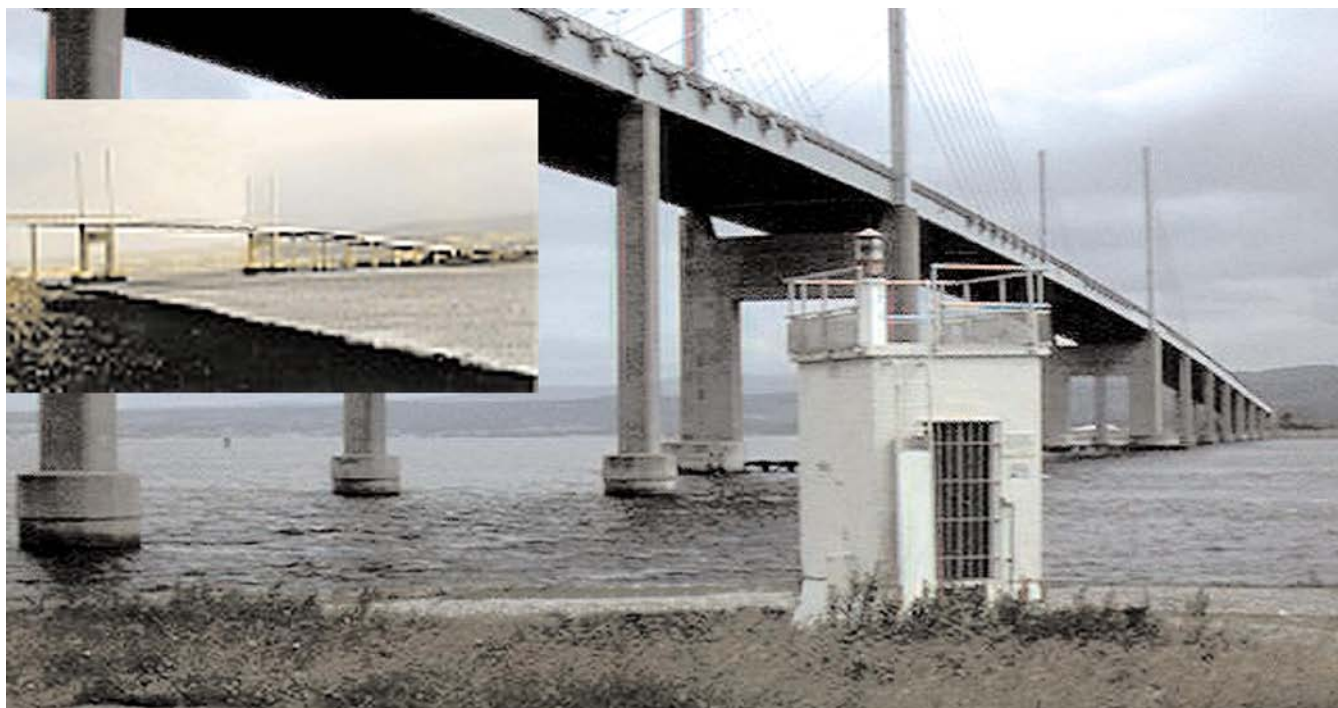
The Kessock Road Bridge
