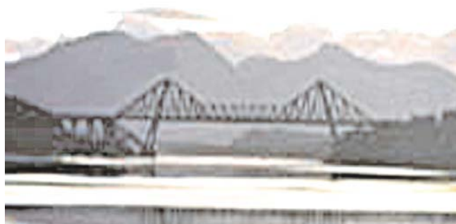
The Connel Bridge
